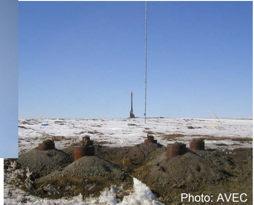
Toksook Bay wind turbine foundation
